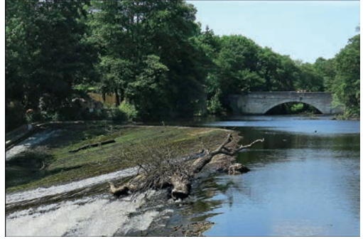
Calver Weir & New Bridge
